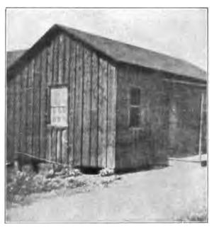
FIG. 21.—AN OLD-STYLE BOARD AND BATTEN 3-ROOM MINER'S COTTAGE STILL IN USE IN AN ISOLATED MINING TOWN OF PENNSYLVANIA.
